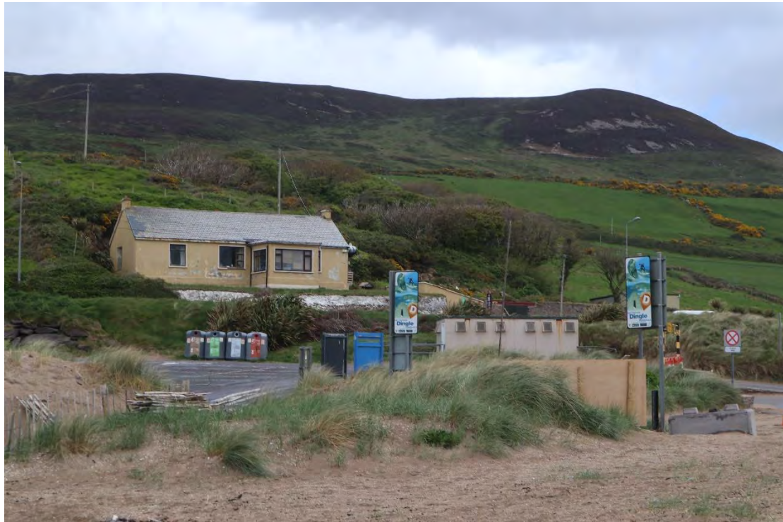
FIGURE 40 INFRASTRUCTURE AT INCH STRAND, CO. KERRY
